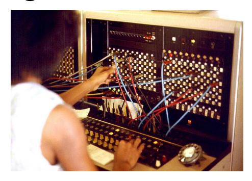
Calls are connected with cord pairs at a telephone switchboard.
